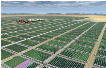
Conceptual artist rendering of a large scale photobioreactor for a coal burning power plant.
