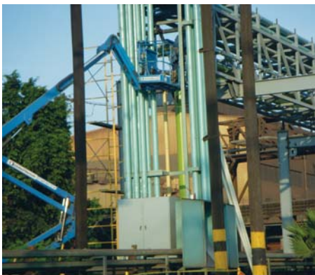
GF Piping Systems' PROGEF Polypropylene Piping System is used for a steel mill's acid recovery and acid regeneration lines.
