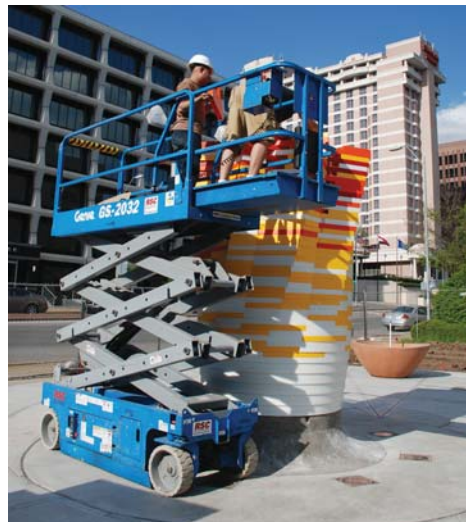
Using a scissor lift on-site, each plastic part could be accessed and mechanically fastened.
