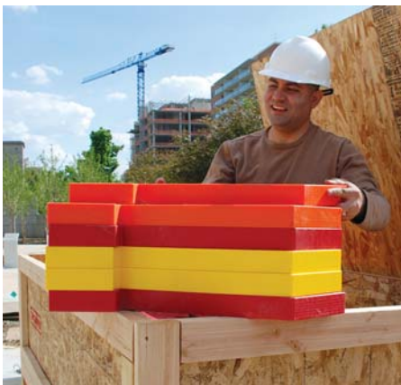
Smith's associate, Burzeen Contractor, organizing HDPE parts for on-site assembly.
