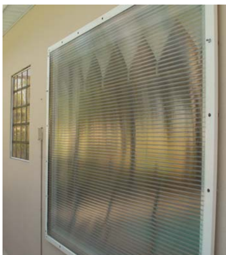
Exterior view of Polygal® Stormguard Florida-approved hurricane system made from high impact 16 mm storm grade (SG) polycarbonate sheet.
