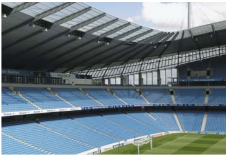
Brett Martin's Marlon CS Longlife profiled polycarbonate sheet was the material of choice for Manchester City's canopy roof.
