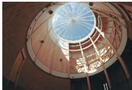
Marlon FS solid polycarbonate created impressive dome rooflights for a football club in Glasgow, Scotland.
