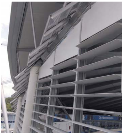
Marlon FSX Longlife solid polycarbonate sheet was the perfect product for Manchester City's canopy roof.
