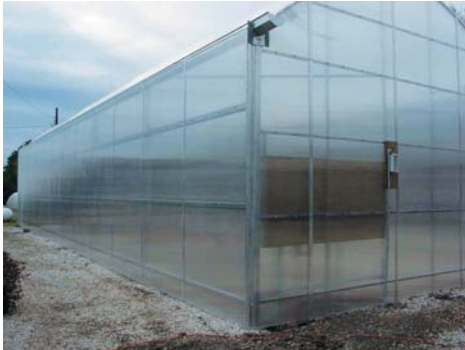
The polycarbonate material chosen for the construction of this greenhouse was Gallina SUV: 8 mm four layers.
