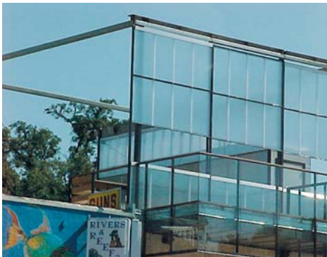
Gallina arcoPlus 684 was used in this large screen for advertising a store in Texas.
