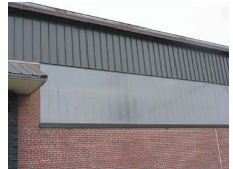
Gallina arcoPlus 323 was the material used for the windows in this manufacturing facility.
